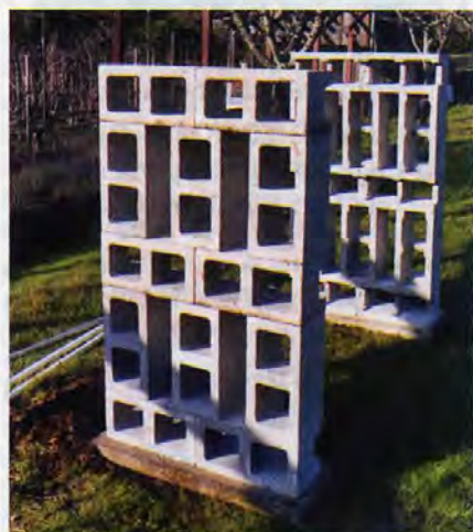
The storage rack main structure: two stacks of concrete blocks.
