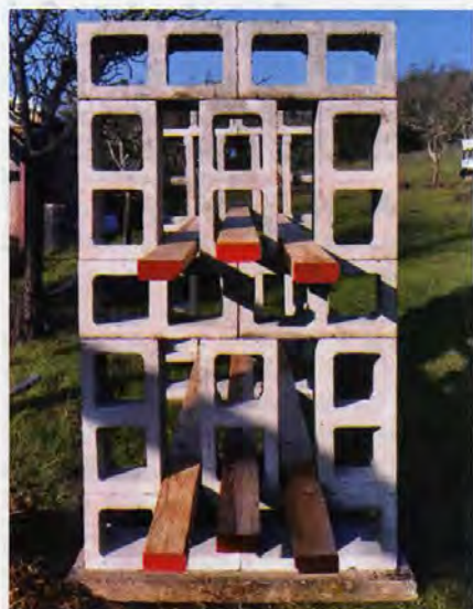
The structure is ready to receive the corrugated sheet metal roofing.
