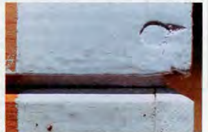
Close-up on a drip edge that separates two hive components. This detail prevents rainwater from penetrating inside the hive by capillary action.
