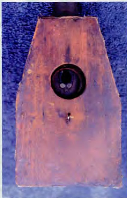
Figure 4. The cleaning cap removed showing the blast tube ready for cleaning.
