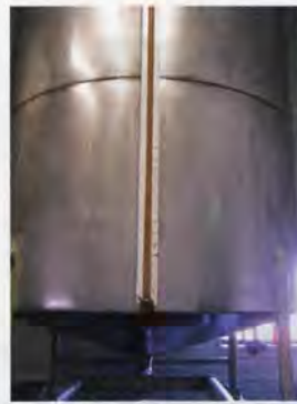
Roscoe's two 2200 gallon storage tanks. Each has a fill tube (inset).
