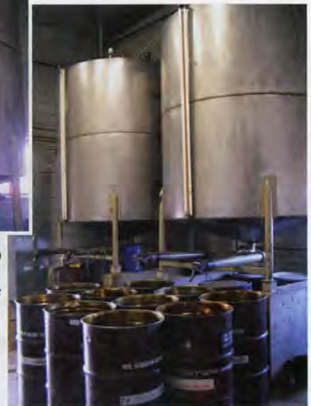
Roscoe's two 2200 gallon storage tanks. Each has a fill tube (inset).
