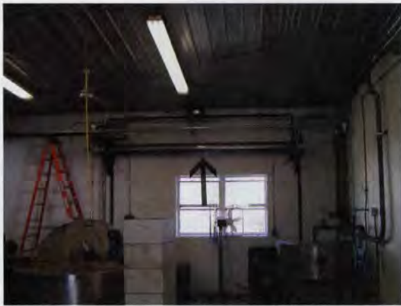
The heat exchanger (arrow) is made of aluminum and filled with hot vegetable oil.
