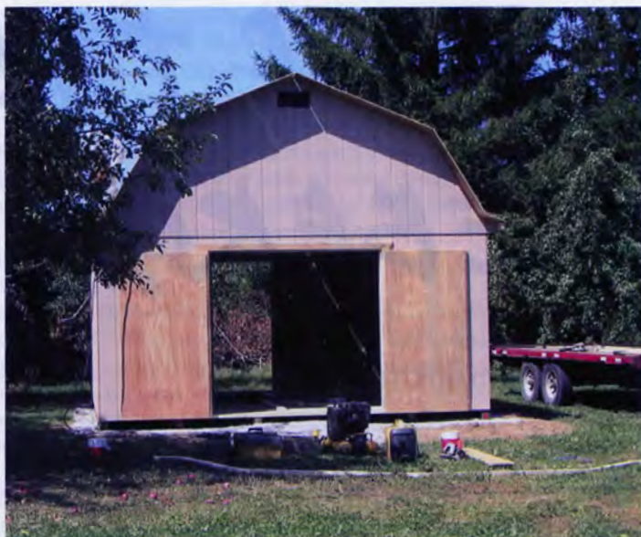
My bee equipment storage barn under construction.
