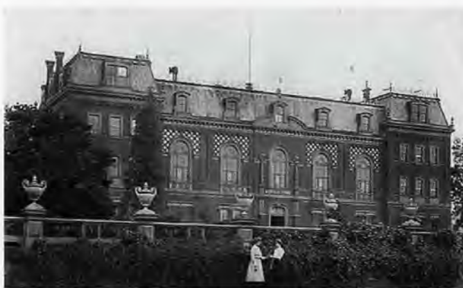
Exterior view of the old Department of Agriculture Building.
