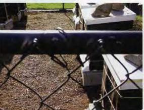
Clips to hold chain link top and bottom.
