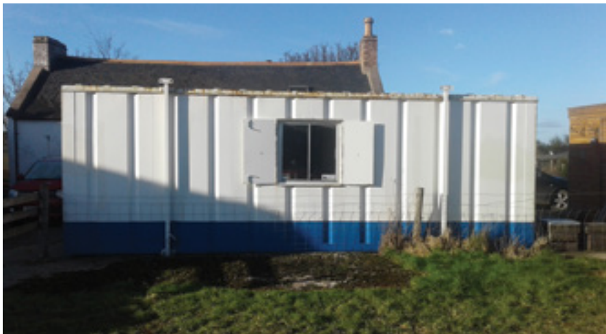
Tony's honey room, a converted shipping container.
