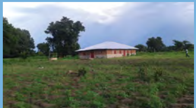
My house built from mud bricks, powered by two 140-watt solar panels and two 150-amp hour batteries.
