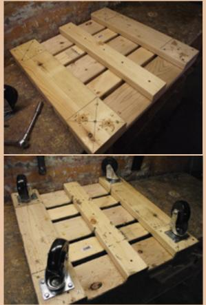
**Step 8:** Position the base so the bottom is up (3 boards). Then add the castors using the lag screws (part #3). Be sure to leave enough room between the lag screws and the ends or sides of the boards to prevent splitting when the castor wheels hit a rough spot which causes stress on the lag screws.
