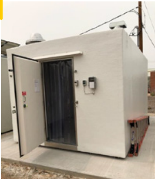
Figure 4. The honey bee cold storage unit (HBCSU), with adjustable ventilation fans, CO 2 sensors and temperature control. Hives inside the cold storage unit. The hives were fitted with individual CO 2 sensors.
