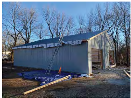
This is how it stands at the time this went to press. Four walls and half a roof. I will take you through the trials and tribulations of the build in the next installment.
