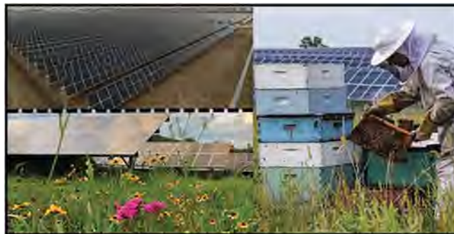
Figure 1. Top left – a conventional solar farm with gravel substrate (Anon 2020). Bottom left – mature pollinator-friendly solar farm. Right – solar farm with a honey bee apiary (photo credit, Dennis Schroeder, National Renewable Energy Laboratory).
